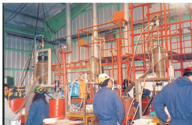
FIG 5 - CMH Imhoflot laboratory pilot plant.
